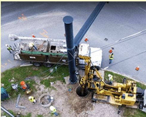
*Installation of a drilled shaft that will support a traffic signal.*
